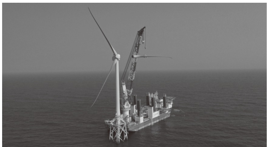
Figure 3 — Offshore Turbine Installation in Progress
