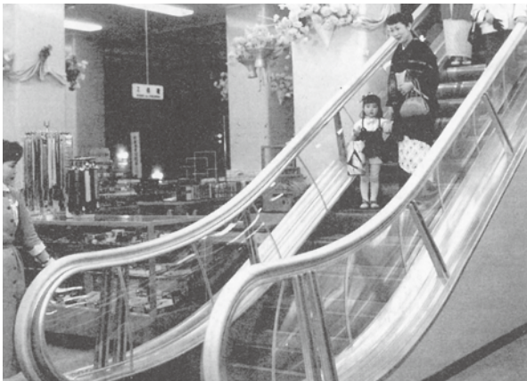
1949 Escalators that became vertical metropolitan pathways
