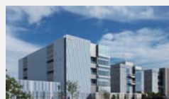
Data center (Okayama No.3 Center)
